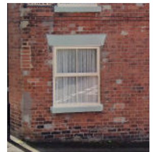
Sashed window with chamfered headers
