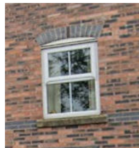
Arched headers with blue engineering brick
